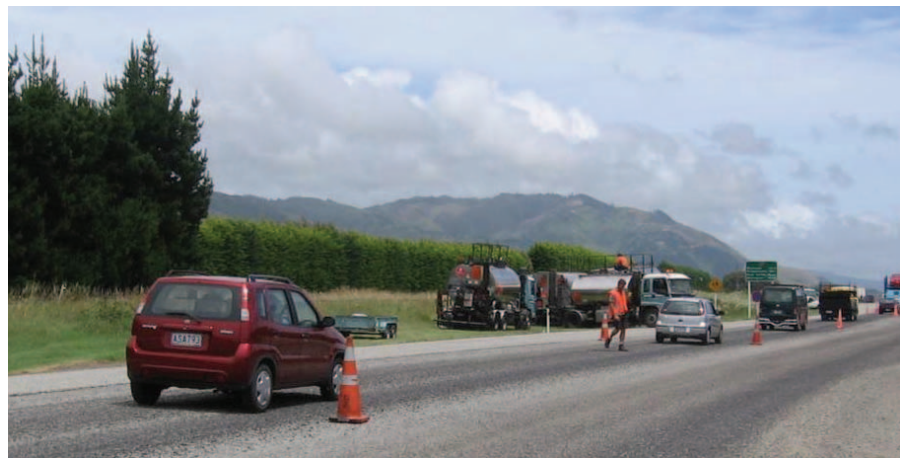
Traffic flowing smoothly during the reseal of SH1, near Otaki.
