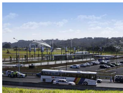
Albany Park and Ride Station
