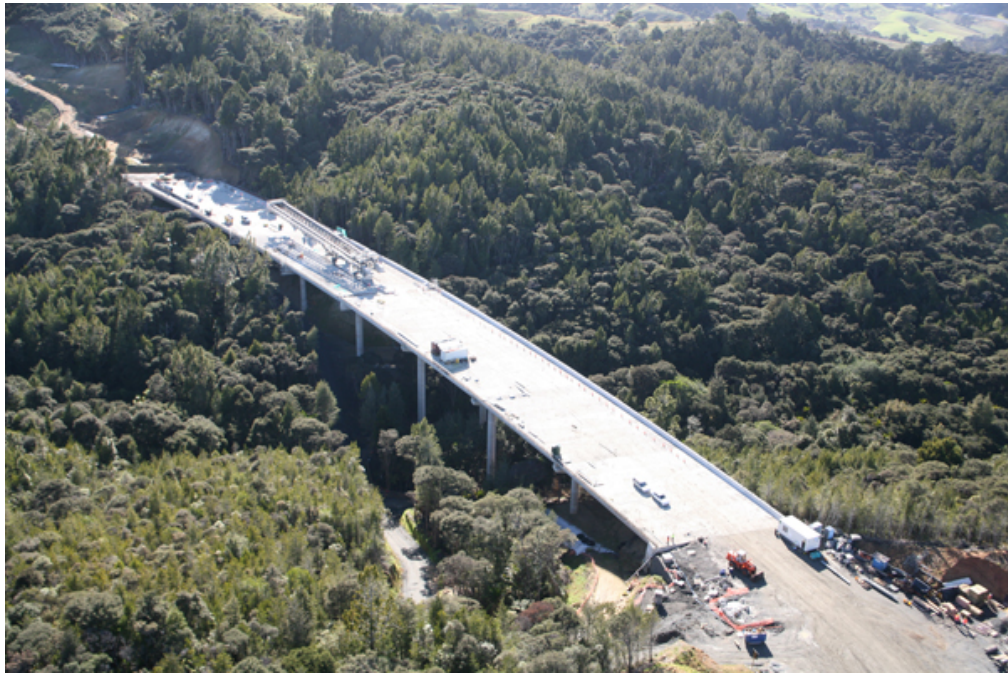
Otanerua Eco Viaduct – example of a context sensitive approach
